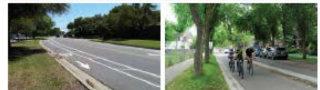
Walking and bicycling facilities (Source: Toole Design Group)
