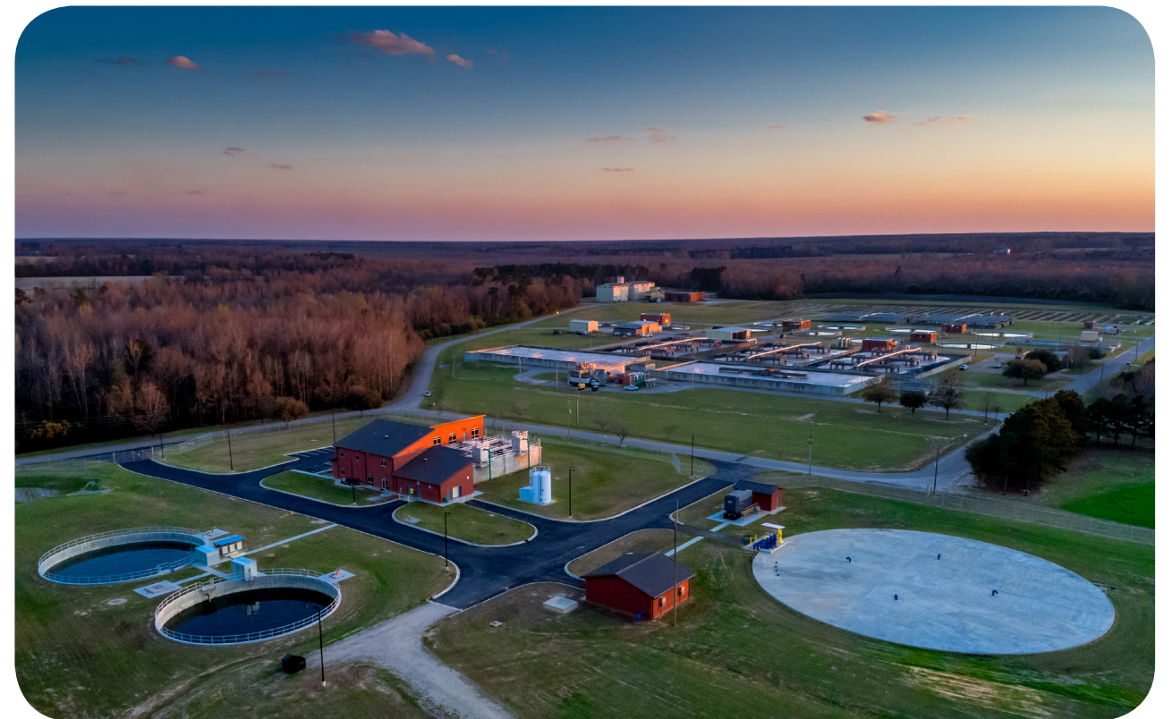
Photo: City of Sumter Wastewater Treatment Plant #6
