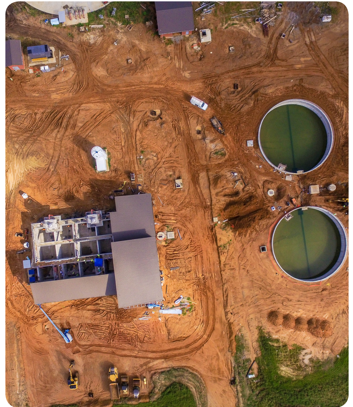
Photo: Construction of Wastewater Treatment Plant #6
