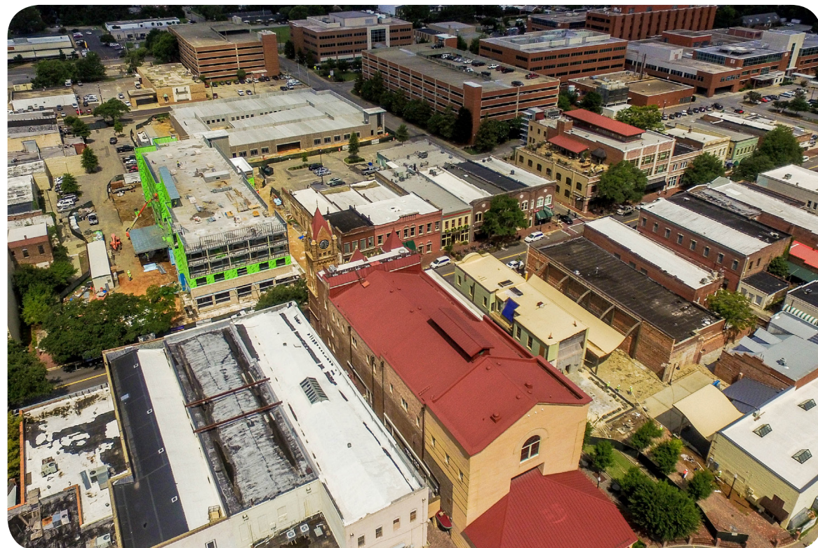
Photo: Construction in Downtown Sumter
